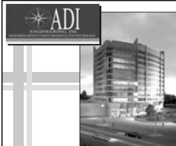
ADJ's professional services were instrumental in the construction of the Zuma Entertainment Center.
