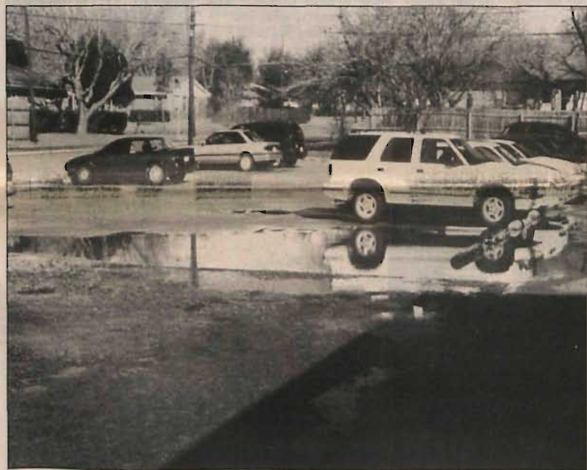
Terrace Elem. will also receive renovated parking areas with better drainage and runoff systems. After rainfall, water collects in the parking lot obstructing the handicapped spaces.
