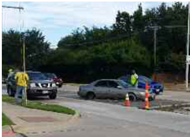
Drivers overlooking barricades can find themselves driving through wet cement. (Image: City of Plano)
